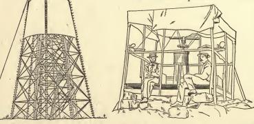
first view the theodolite is not visible, but in the second it is seen mounted upon the tripod. In both views heliotropes for flashing to the adjacent stations may be distinguished. Detailed information regarding the erection of towers will be found in the Report of U. S. Coast and Geodetic Survey for 1882, pages 199–208.
